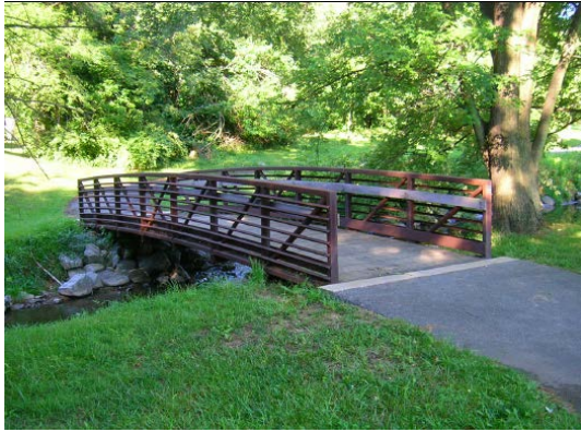
Carroll Creek Elevated Footpath
